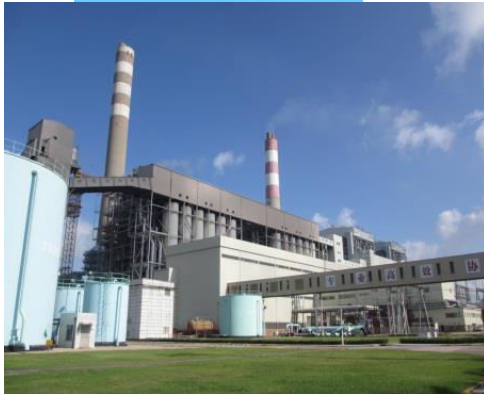
Chinese plant Z1&Z2 700MW x 2 (2013) 541/568°C
