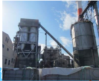
Domestic plant J525MW x 1 (2012) 543°C
