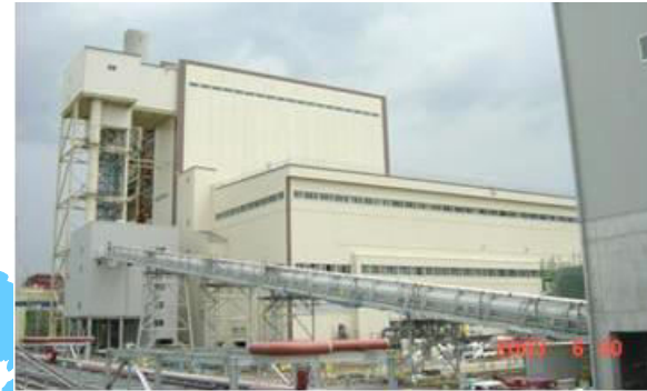
Domestic plant H5 600MW x 1 (2014) 604/602°C
