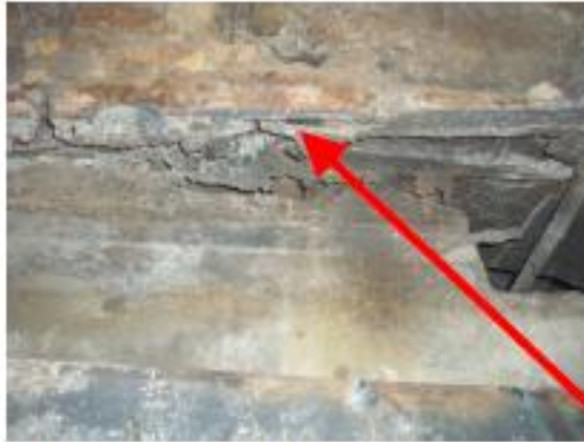
Large cracks in Bottom Hopper Seal Trough seal plates and trough connections to hoppers
