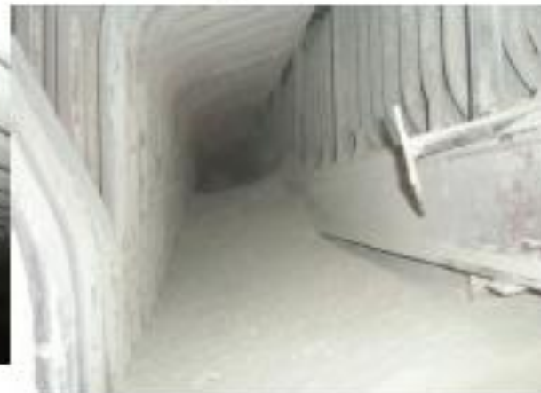
Large cracks in Bottom Hopper Seal Trough seal plates and trough connections to hoppers
