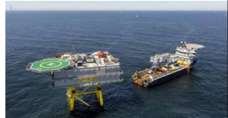
New build project
