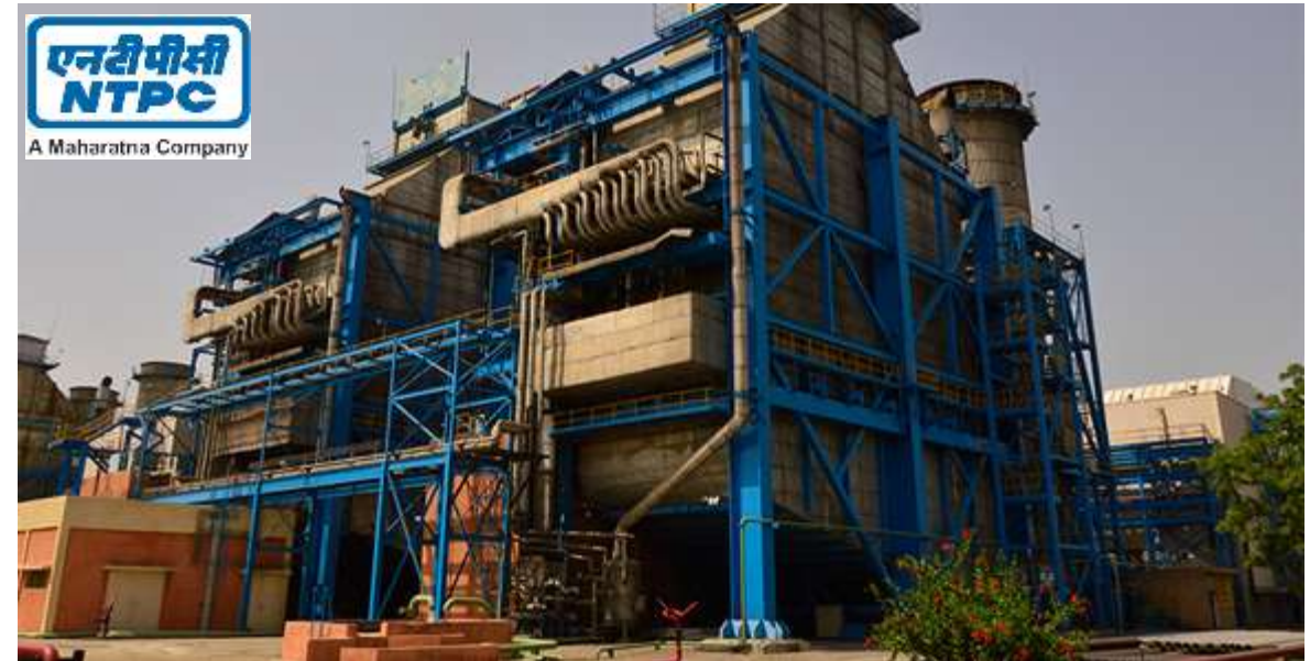
NTPC Dadri Stage II – Unit #6 490 MW
