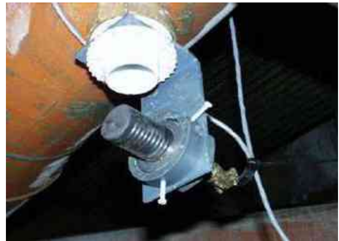
FIGURE 5 - View of Probe Installed in Tap
