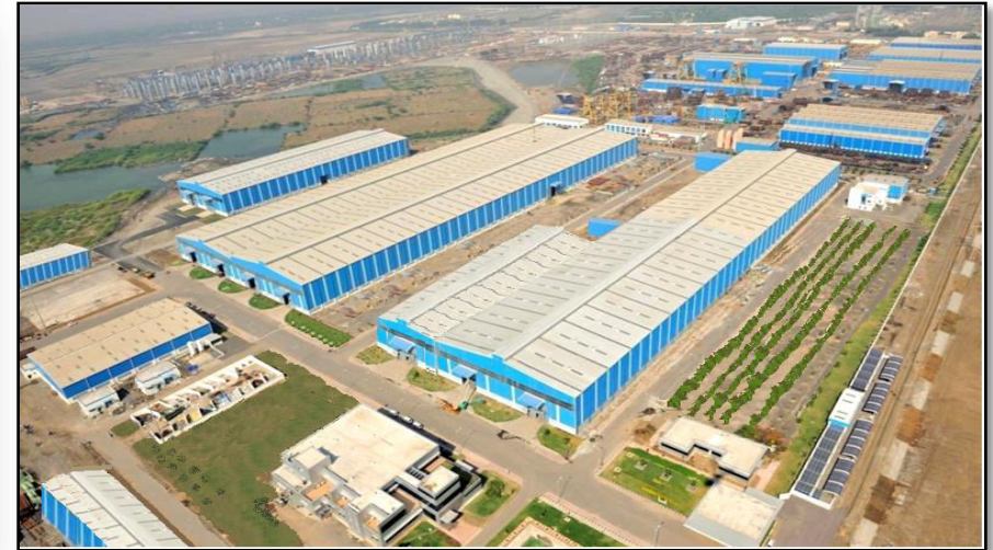
Manufacturing Facility, Hazira
