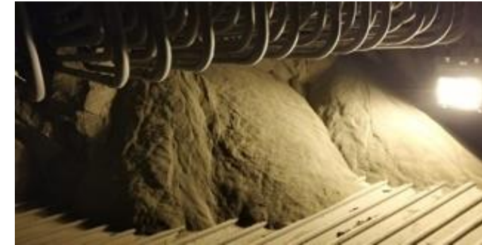
Ash Deposition at Low Loads
