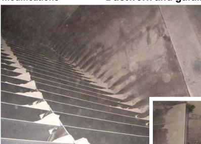
Guide vane level in duct section between air heater and ESP
