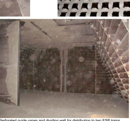
Perforated guide vanes and dividing wall for distribution to two ESP trains
