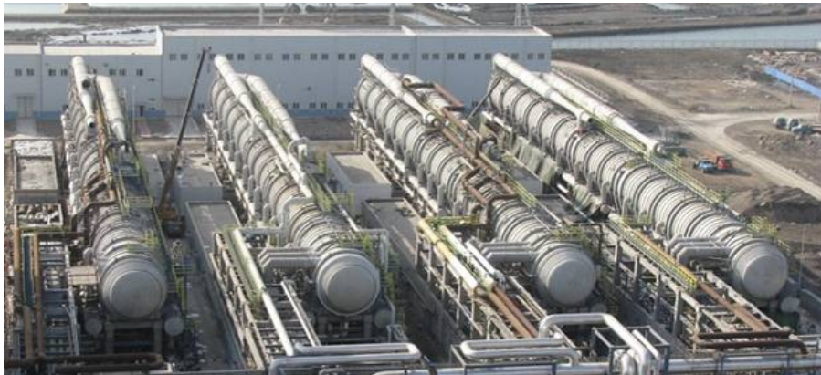
Tianjin, 200,000 m 3 /day China's largest MED desalination facility
