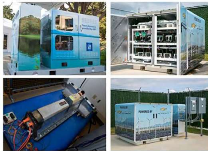
Figure 4.4: GM-ABB Second-Life Electric Vehicle Battery Applications
