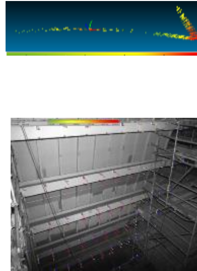
Coal bunker when filled
